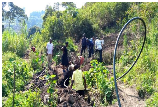
Ongoing trench excavation and pipe laying for Ruheza GFS Implementation
