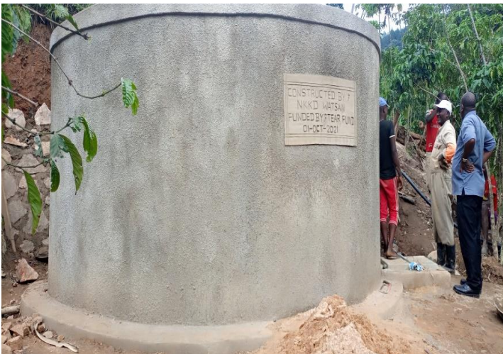
A 20m 3 Reservoir tank, behind which a retaining wall is under construction
