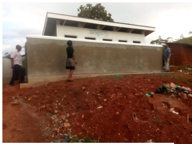
A lined five stance pit latrine with a urinal for boys newly constructed by NKKD WATSAN at Bwanga SSS
