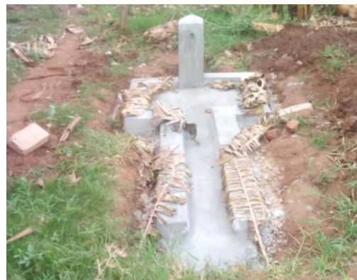
One of the constructed tap stands, Bwanga Hill Project.
