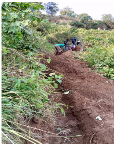
Ongoing trench excavation and pipe laying for Ruheza GFS Implementation
