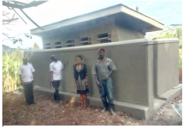
A lined five stance pit latrine with a urinal recently constructed NKKD WATSAN at Bwanga church
