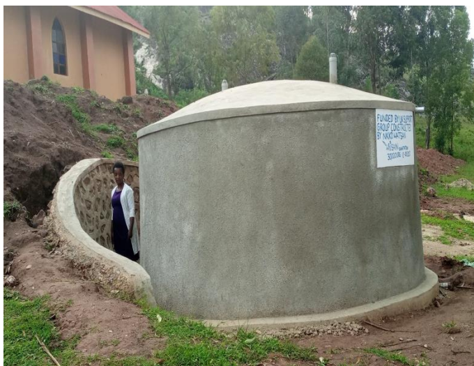
A 30m 3 Rain Water Harvesting Tank constructed at Bwanga Church by NKKD WATSAN to be used by student boys and resident staff at Bwanga SSS
