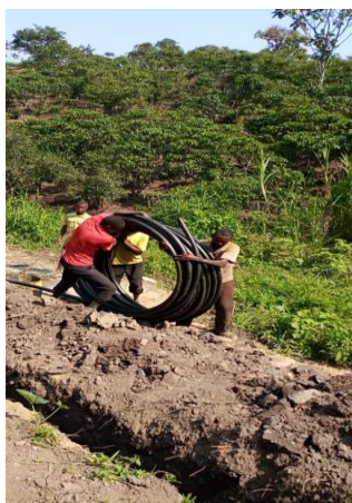
Ongoing trench excavation and pipe laying for Ruheza GFS Implementation
