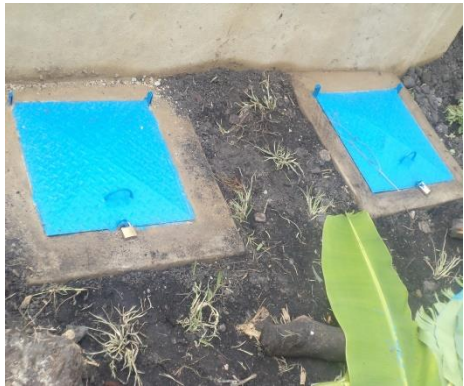
Constructed valve boxes at Kiringa water source
