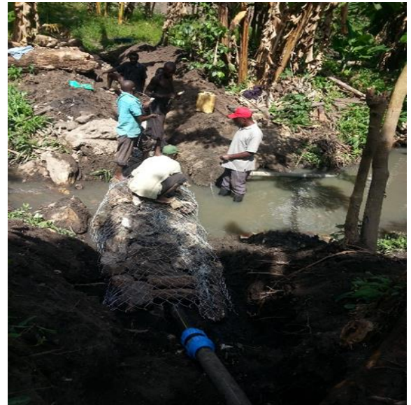
A pipe being protected with chain link at Karerema GFS
