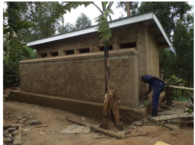
A 6 stance pit latrine for girls under construction
