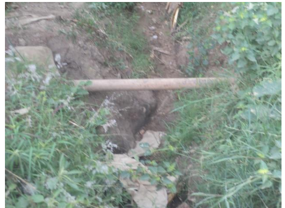
Constructed stream crossing across a valley during Kiringa GFS pipe laying
