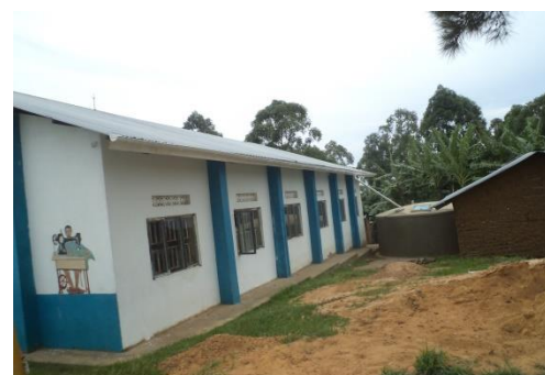
Constructed 30m 3 Rainwater harvesting tank, located between 2 buildings at Rwerere CDC
