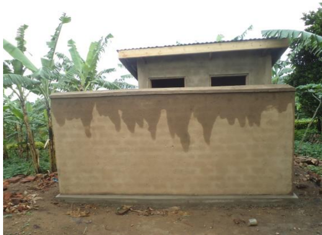
2 stance Pit latrine with a urinal under construction at Nyarugunda Parish
