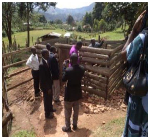
One of the tapstands constructed and finished in Omukyishanda village
