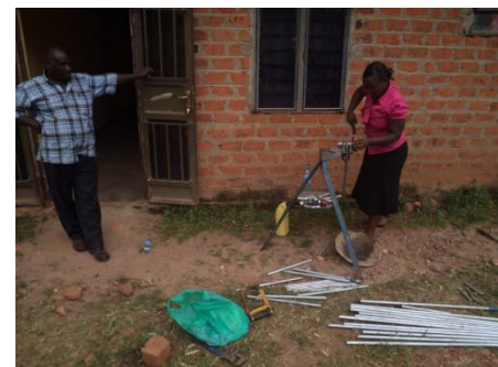
Pipe threading ready for tapstand construction
