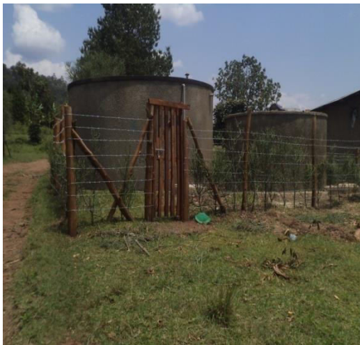
2 tanks at Katunga fenced and finished
