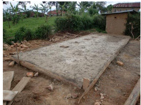
Reinforced concrete base slab of latrine
