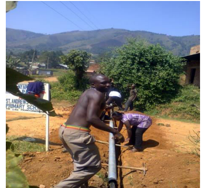
One of the road crossings under construction
